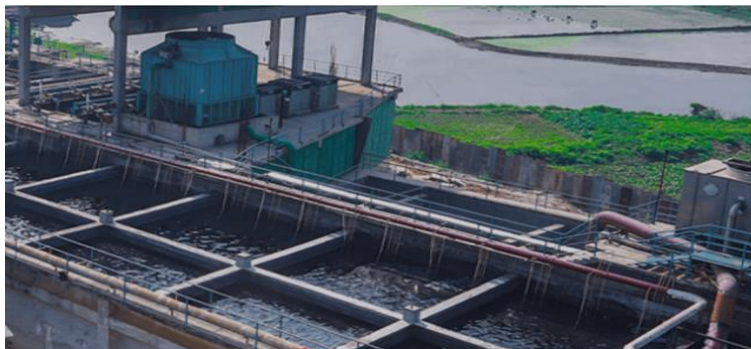
Figure 1: ETP Plant with MBR technology used in Tamishna group at Tongi, Dhaka, Bangladesh.
